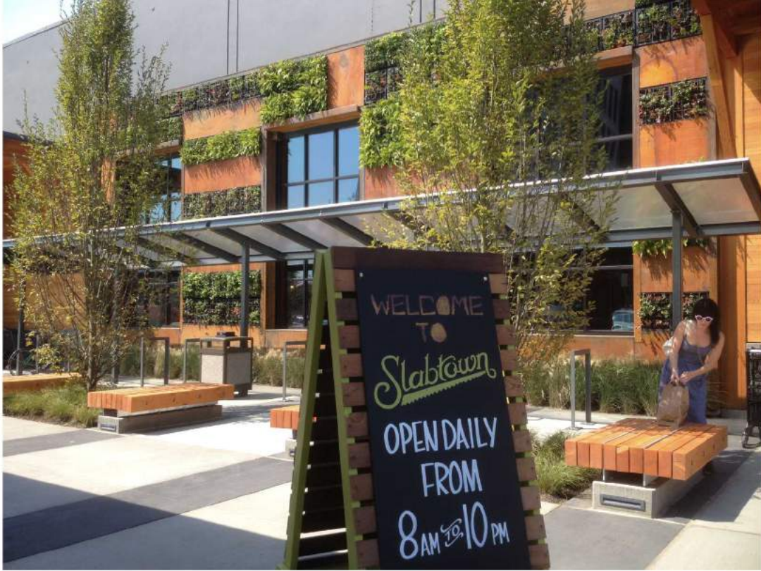
A vegetation pocket wall on an old industrial building made into a New Seasons grocery in Portland, OR. (See also "Rusted Metal Siding")
