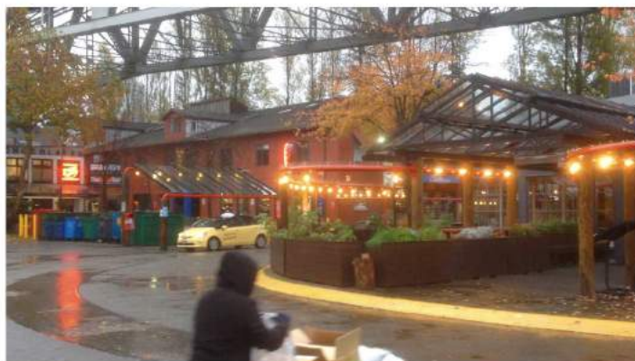
The buildings at Granville Island in Vancouver BC are quite simple and industrial, but they form a delightful series of human-scaled places.
