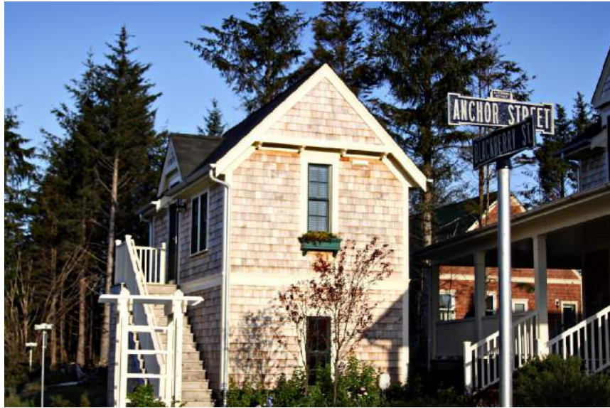
Good downspout locations in Seabrook, Washington include corners and natural breaks in the elevation. Downspouts are straight and clean in all cases..
