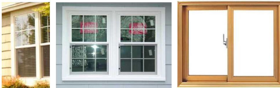
Things to avoid in windows: shallow reveals, plastic clip-in muntins, and windows that are too wide in relation to height.
