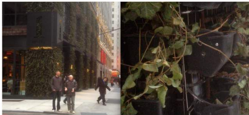
A system of vegetation pockets at a hotel in New York. Small pots are held on a meshwork. The drip irrigation system is visible at right (black tubes).
